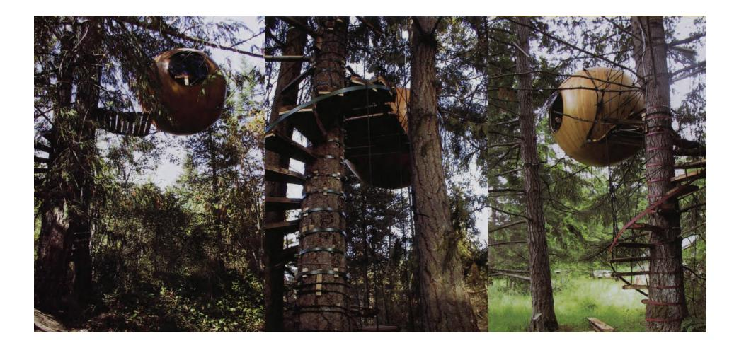
The house is supported by a set of ropes attached to separate trees that evenly distributed the 500 pound load. If one rope breaks the rest of the ropes will still support it.
